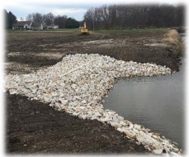
Grade Control Structure
