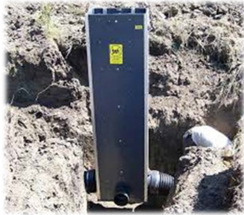
Water Control Structure
