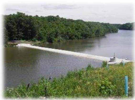
Low-flow/in-lake dam; Otter Lake, Illinois
